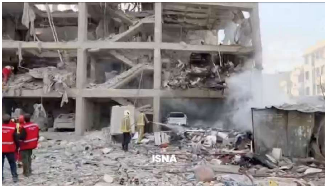
Still from a video showing rescue workers in front of the Number 12 residential building that was likely directly hit. © ISNA
