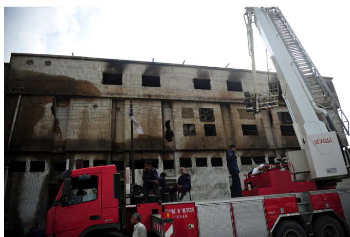
↑ Workers burned to death or suffocated in the massive blaze that engulfed Ali Enterprises clothing factory in Karachi, Pakistan. Photo: Getty Images
