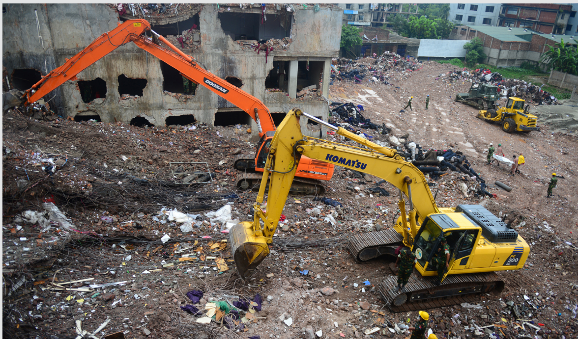
↑ Heavy machinery clears the debris on the site of the collapsed Rana Plaza garment building on the outskirts of Dhaka. Photo: Getty Images
