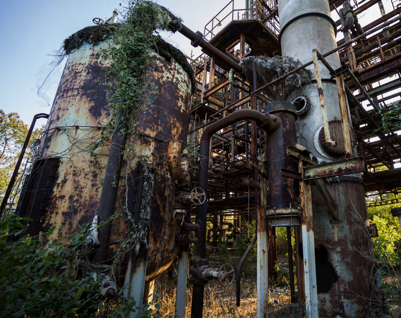
The processing plant. 2014 © Giles Clark
