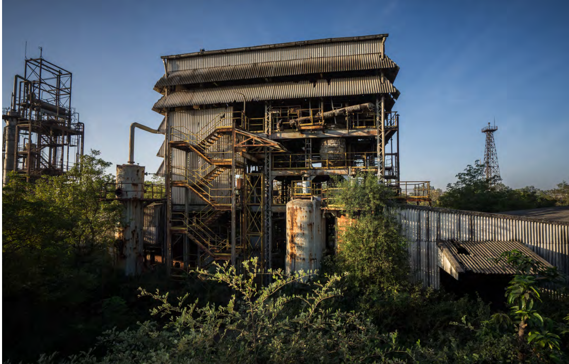
UC chemical processing area with flare tower © Giles Clark 2014
