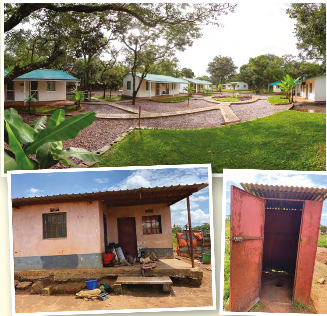
© ↑ Units built near Kakula to provide on-site accommodations for Kamo's employees and contractors © Ivanhoe Mines Ltd. (top); Resettlement houses and bathroom built in Muvunda where Kamo resettled communities who used to live on the surface area of the Kakula Mine, 26 February 2022 © Amnesty International (photographer: Jean-Mobert Senga)
