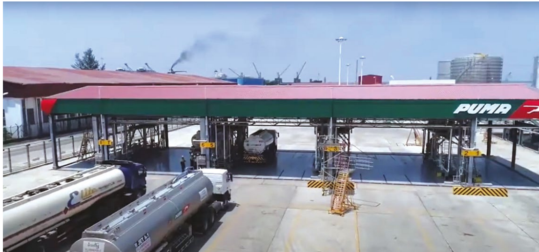
PEAS terminal, Thilawa port: The PEAS terminal has a loading bay where tanker trucks are loaded with the aviation fuel that is distributed to storage facilities across the country. 349
