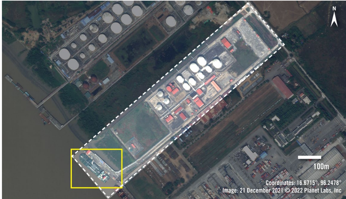
Puma Energy Terminal, Thilawa, Myanmar: Satellite imagery from 21 December 2021 shows a ship at the Puma Energy berth in Thilawa, Myanmar. Vessel tracking data documented the vessel, Synergy, at Thilawa around the time the image was taken. The length, breadth (154m x 36m) and colours of the ship in the image match that of the Synergy.
