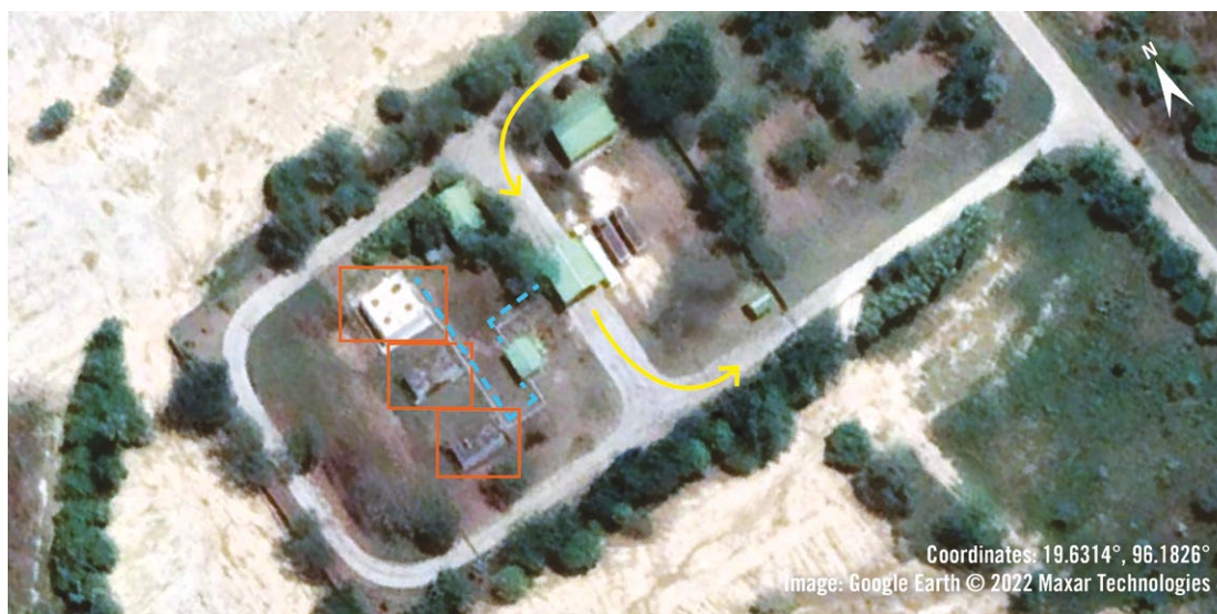
Nay Pyi Taw, Myanmar: Satellite imagery shows the fuel storage facility adjacent to the Nay Pyi Taw military base. The fuel storage tanks are highlighted in orange squares, pipes are traced with a blue dotted line and roadway design shown with yellow arrows.
