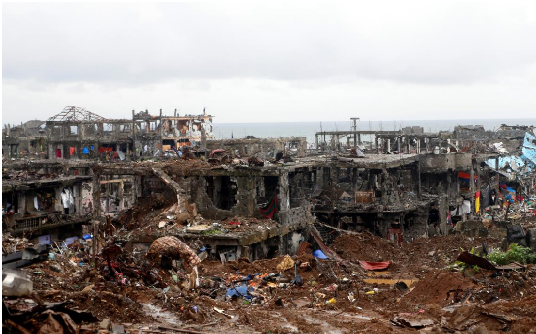
A general view of the damage in the eastern part of Marawi city where the fighting was mostly concentrated, 17 October 2017. © Jeffrey Maitem/Anadolu Agency/Getty Images
