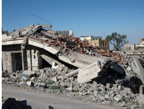
A destroyed house, Sa'dah, Yemen, March 2010. The graffiti reads “This is the help Yemen gets from America” © Private
