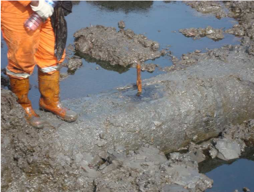
Leaking pipeline near Bodo, 30 June 2012: A wooden stick was hammered in to the leak point to prevent further spillage. © CEHRD
