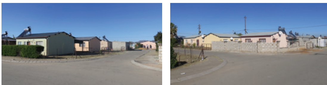
Houses built before 1994. Some have been refurbished by recent owners. © Amnesty International
