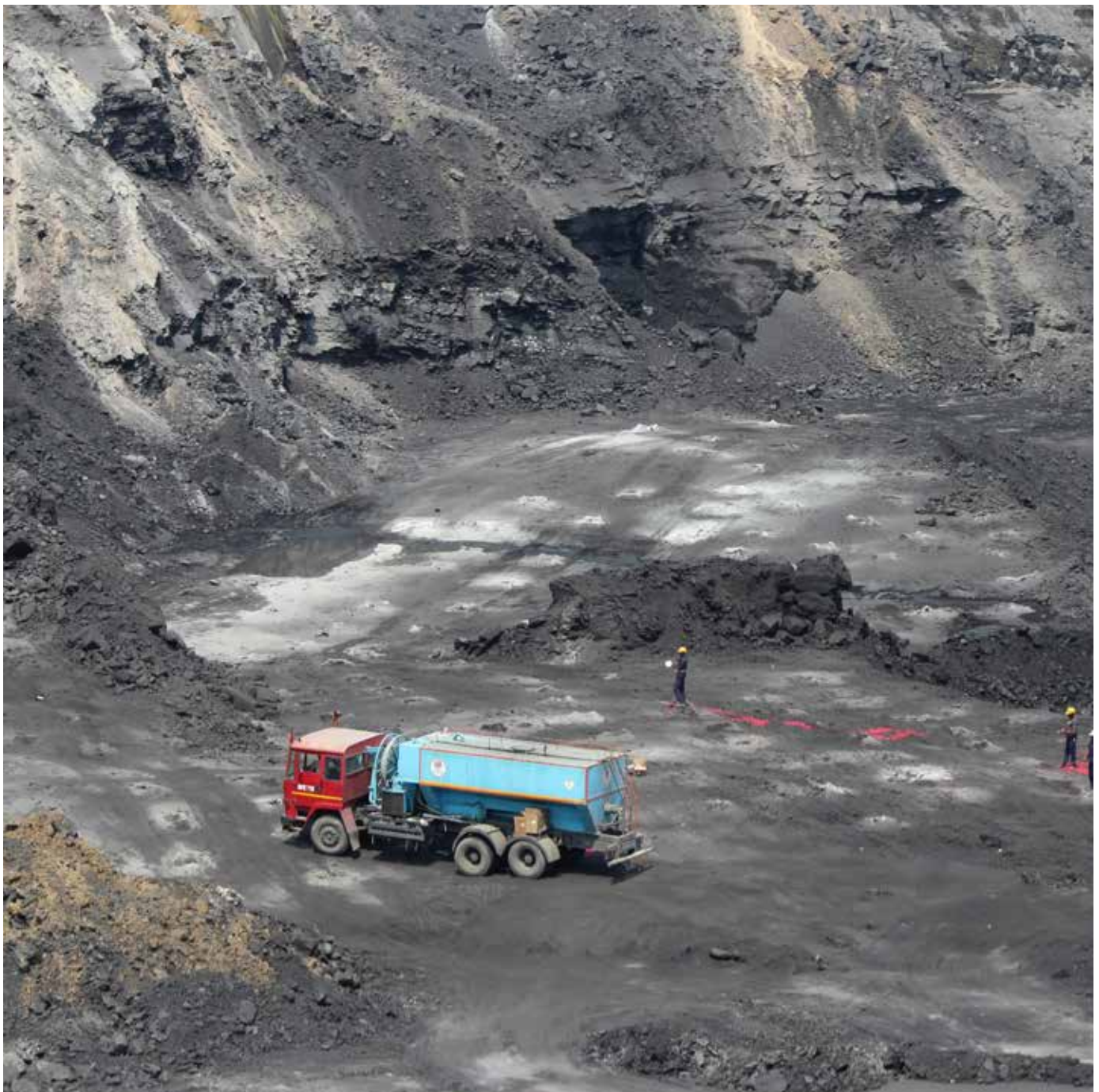
An SECL engineer marks the spot where blasting will take place, Barpali village, April 2014. © Amnesty International India
